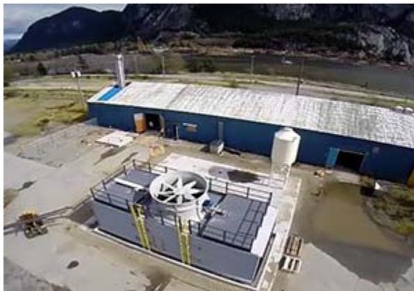
A large fan pulls CO<sub>2</sub> from the air at a pilot facility operated by Carbon Engineering in British Columbia.
